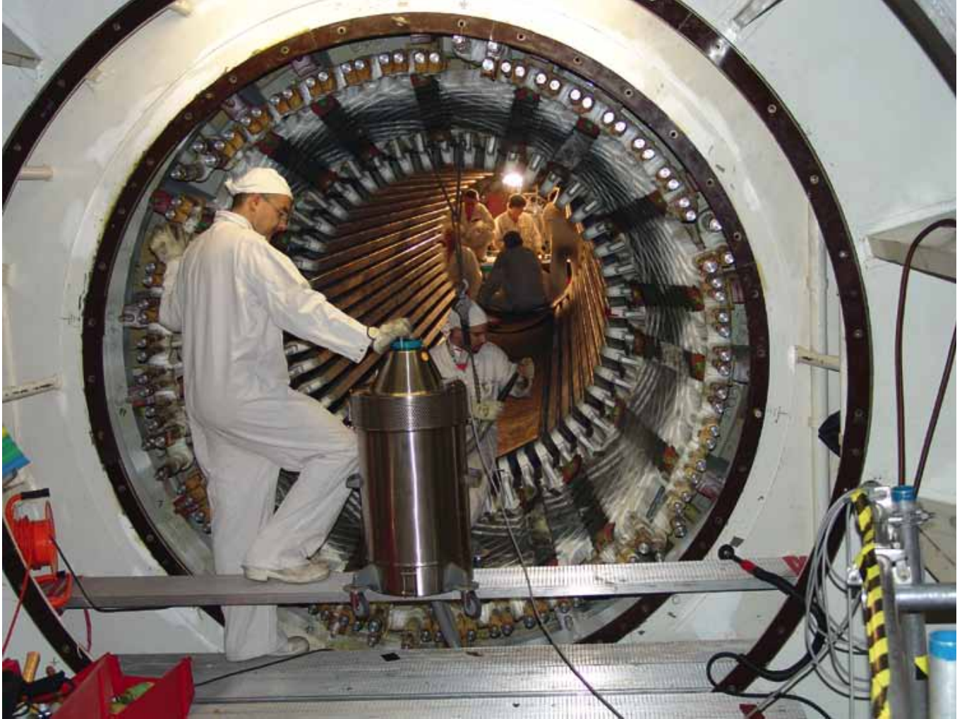
When the rotor is dismantled, a look into the generator shows the winding head with the connections for the water cooling system.
