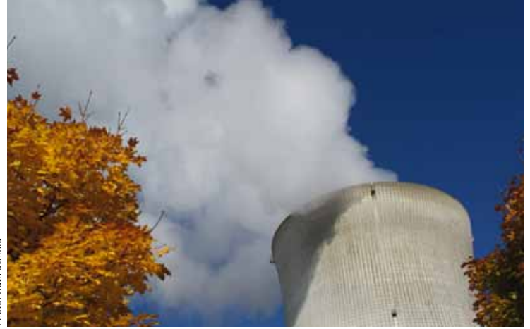
Pure water vapor comes out of the cooling tower.
